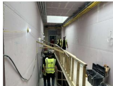
Block 1 FF Hallway
